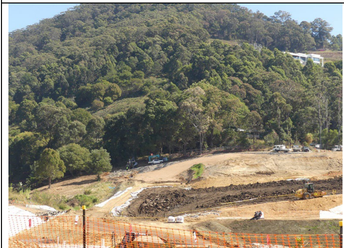
More mountains of soil being removed.
