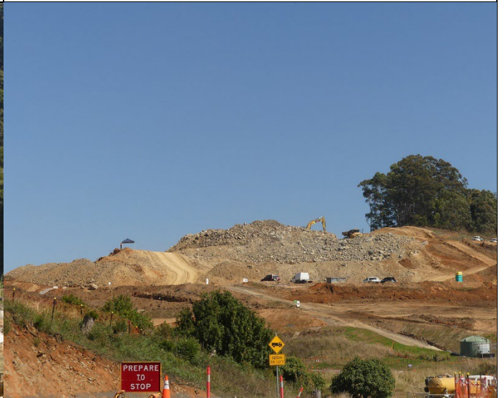
Mountains of soil being removed.
