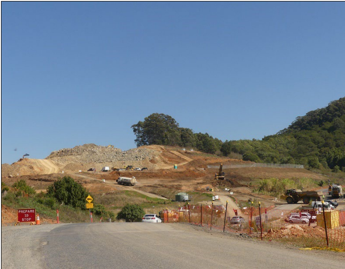
Bruxner Park Road – construction work on the hill.
