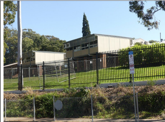
The James Small Drive – back of the school, with a playground fenced off from the construction zone.
