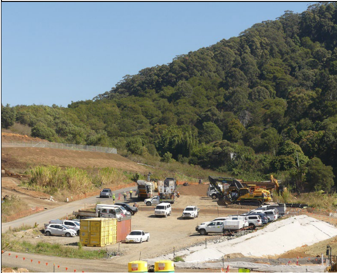
Land cleared below the bushes and construction work underway.
