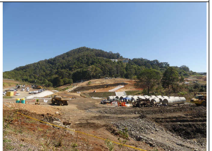
Pipes at the foot of the trees, ready to be laid.
