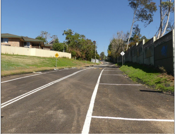
A small number of new marked parking areas on School Road off Russ Hammond Drive.
