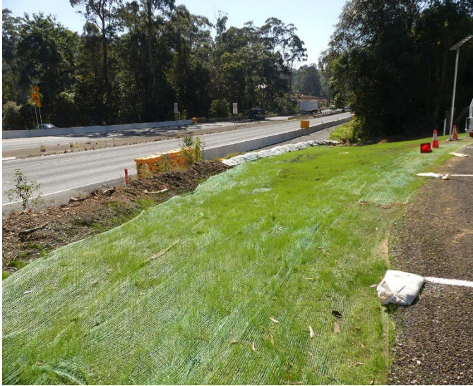
The now grassed in old School Road entry from the highway.
