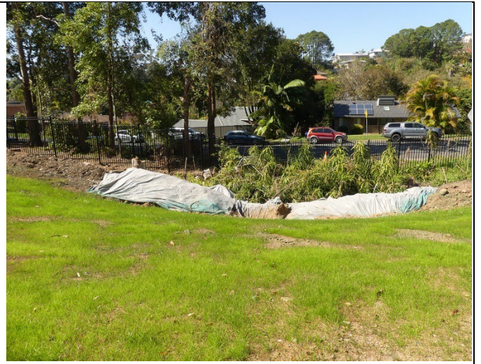
The bottom playground area with construction drainage.
