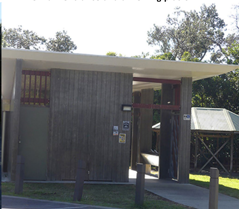
The modern facilities and covered areas
